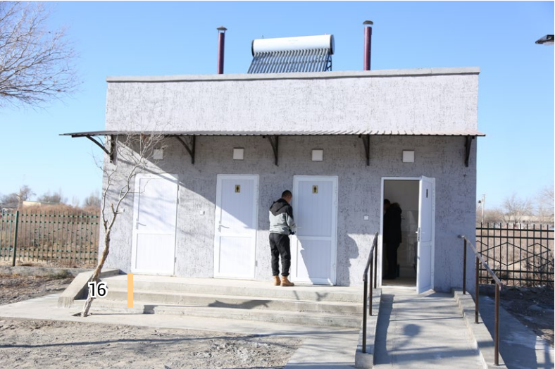
Photo 10. Sanitation facility at the Rural Health Care Point 'Suwenli', Kungrad district.
